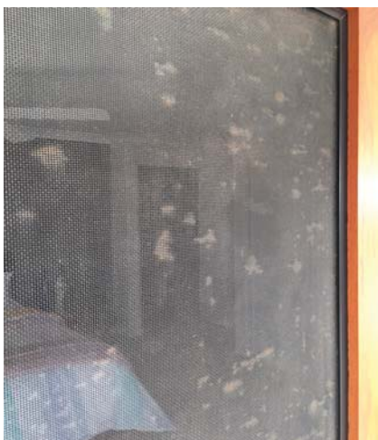
Dirt build up on a woven S.S. mesh
